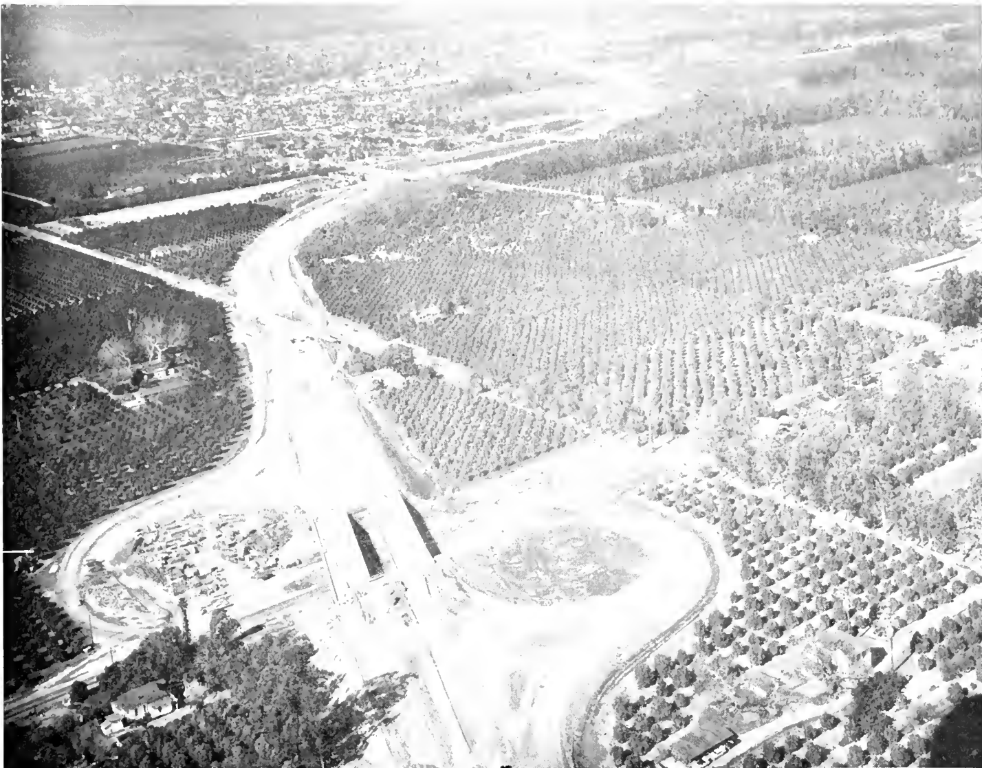
Looking northerly on Santa Ana Freeway from Tustin Avenue to First Street. The completed Route 2/43 separation structure is shown in foreground.
